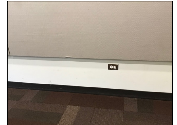
IS 92 Some of these showing scuff marks and damage
